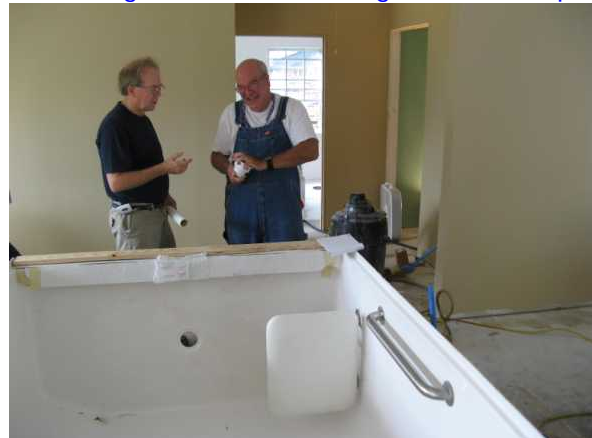
Planning the next move at our project
