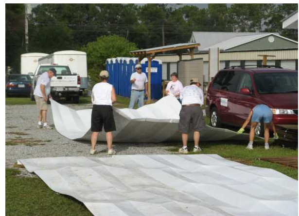
Building additional housing at PDA camp
