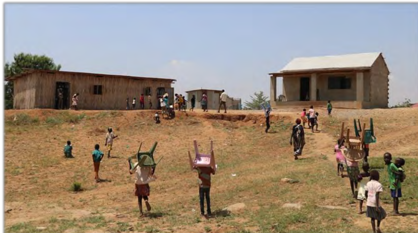
The two classrooms on the left built by committed parents
