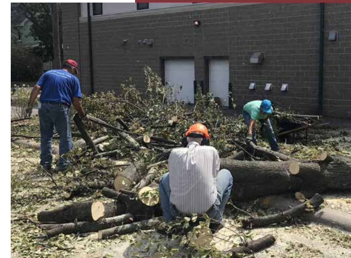
Local volunteers cleared debris from First Presbyterian Church of Cedar Rapids.
